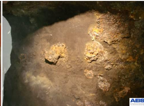
Figure 2: Deposits on the inside surface (waterside) of the fractured segment
