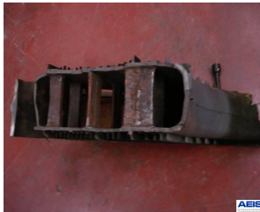
Figure 5 Restraining Baffles Behind Crown
