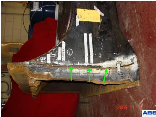
Figure 1: The main crack
