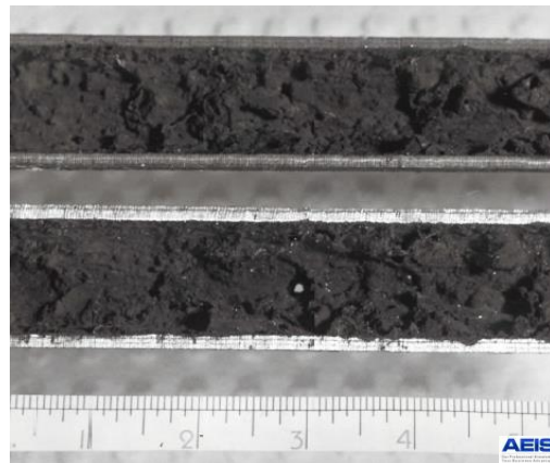
Fig 3 Inside surface of the pipe
